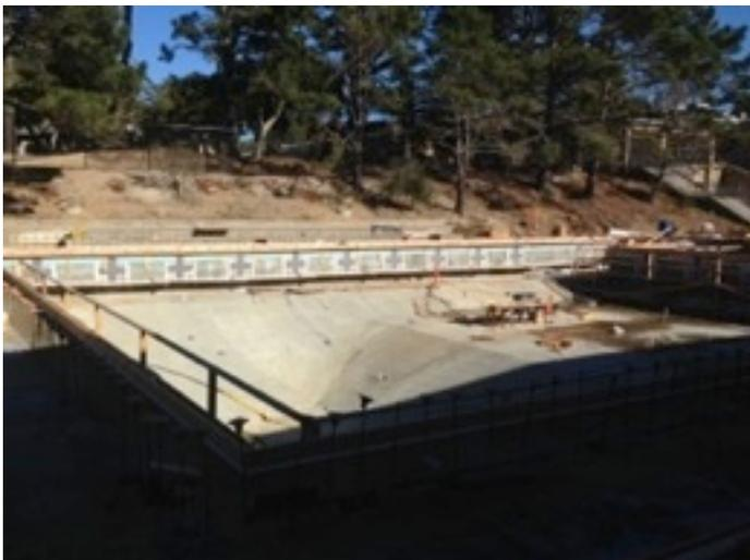
View to L shows diving well going to depth of 13 ft. Far embankment still has old cement bleacher area from old pool deck design. Ten competition 25-yard lanes will vary in depth from 4'9" to 13' with starting blocks installed on wall nearest gym. These photos were taken in October. Page 1 shows pool filled, lights on.
